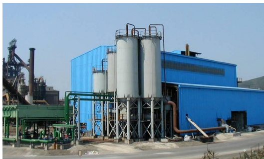
RedIron Plant at Lucchini SpA, Piombino, Italy
