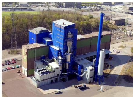
ArcelorMittal Woierer By-Products Recycling S.A., Differdange, Luxembourg
